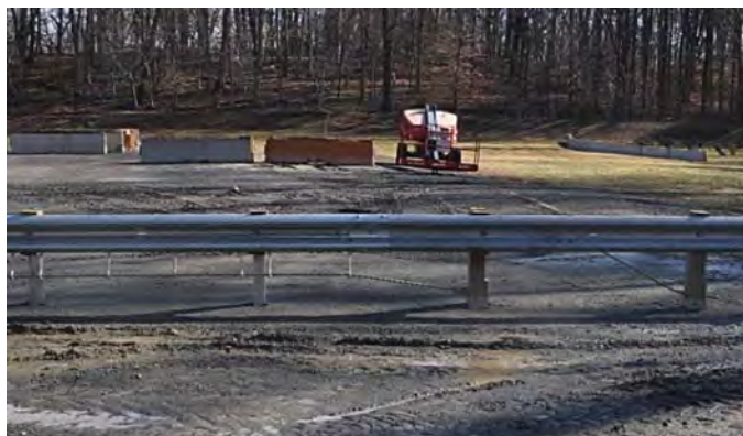
Front view of the top and bottom cables on the side road. Lower cable anchored with a bearing plate.
