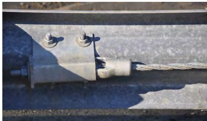
Back view of the top cables on the side road using half of a standard anchor bracket.
